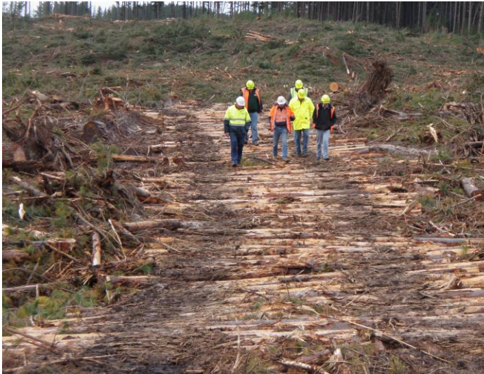
Cording across a wet low-lying area on a major forwarding track
